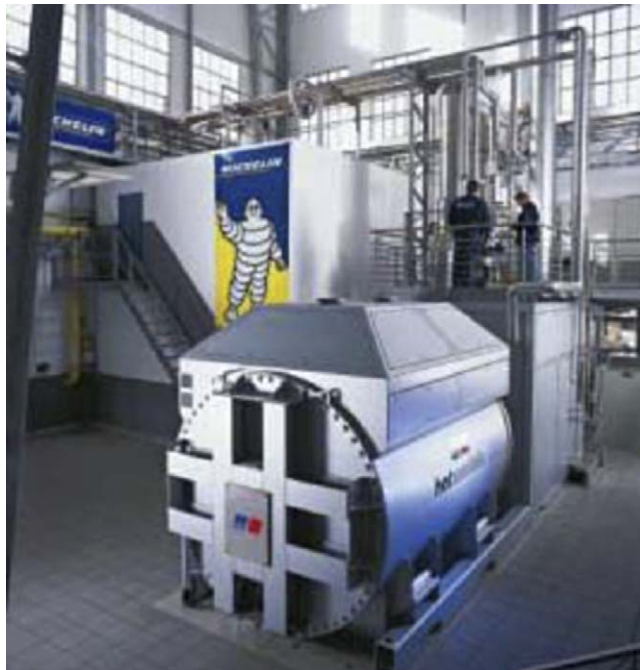
Fig. 9. MTU's hot module is in operation at a factory: an indoor 250 kW unit operating in a industrial environment.
